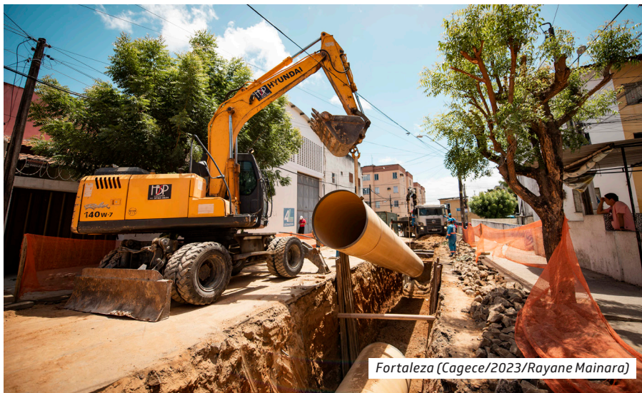
Figure 4: Construction work for the implementation of Conventional Sewerage
