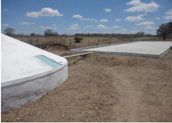
52-thousand-liter sidewalk cistern
